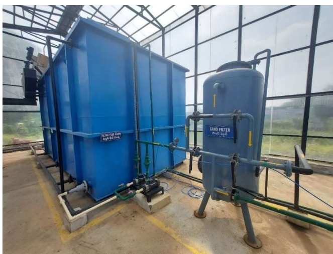
Figure 12: The image here shows the MBBR's main treatment module from front side view
