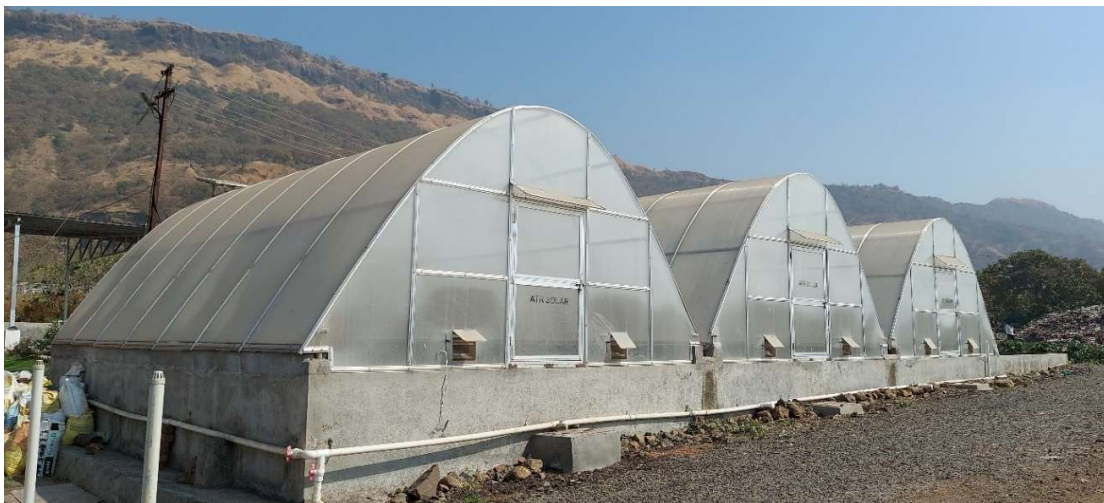
Figure 4: The regulated solar-dryer based drying beds at Satara FSTP
